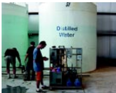
Norland crew working on ozonation equipment in Blue Valley's pre-treatment area.
